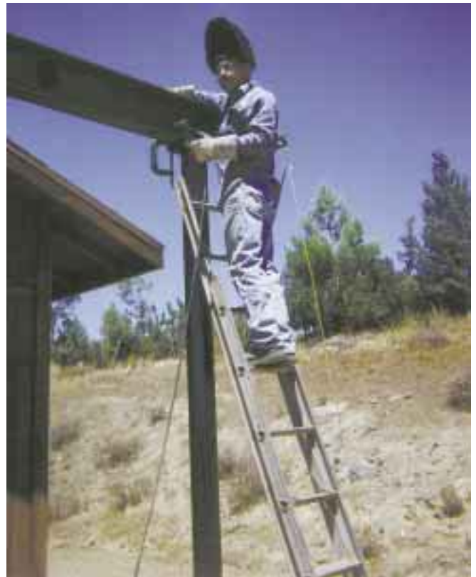
Welding the newly placed I-beam.
