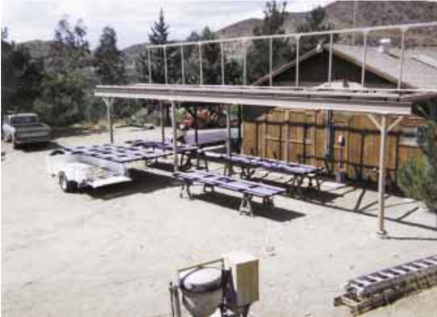
The subarrays all wired up and mounted on the frames, which are primed, painted, and ready for installation.
